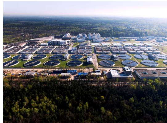
Water and Sewerage plant, Warsaw
